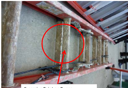
Excessive Paint on Rungs
