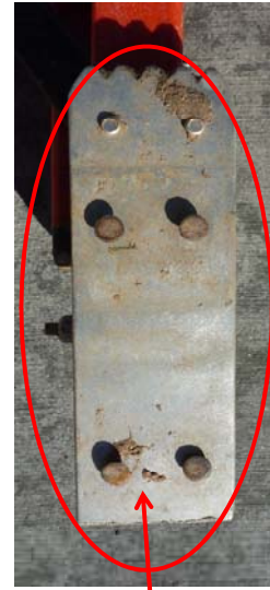
Missing Rubber on Foot
