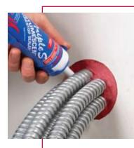
Premium grade, water-based firestop caulk featuring STI's patented two-stage intumescent technology. The perfect choice for the broadest array of combustible and non-combustible electrical penetrants requiring a permanent, durable seal.
