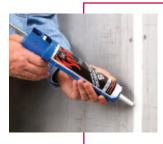
Flexible Firestop Protection for Fire Rated Joints.
