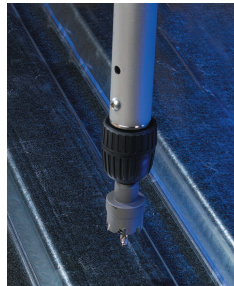
2. Drill Deck Holes
