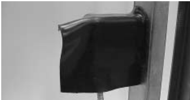
Step 3: Starting at top, align to front edge of box and overlap onto the stud 1/2 inch (13 mm).
