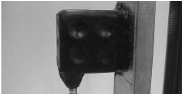
Step 6: Trim excess putty from corners and apply it to conduit fittings or cables connected to the box. Ensure pad is pressed firmly to surface of top, back, bottom, and side of box.
