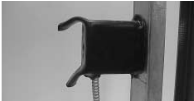
Step 5: Extra putty will pleat at corners after pad has been applied to surface of box.
