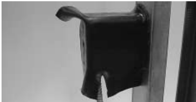
Step 4: Adhere remaining pad to box and cut to provide a snug fit around conduits or cables.
