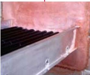
Strong, lightweight, cementitious mortar mixes with water to seal medium to large openings typically used for cable trays or banks of conduits.
