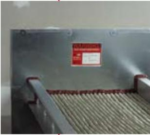
Lightweight, easily fabricated panels surface mount to walls and floors to provide a neat, clean firestop seal for medium to large openings typically used for cable trays, bus ducts, and conduit banks.
