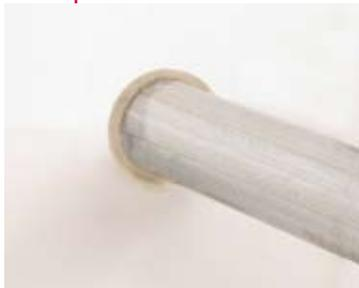
A 100% silicone firestop caulk engineered to rapidly cure and resist washout when used in exposed conditions.
