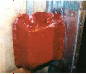
Externally applied to switch and receptacle boxes, pads are UL Tested and Classified to permit larger boxes and reduced spacing in gypsum board walls.
