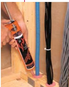
Standard grade, water-based firestop caulk engineered to address most common combustible and non-combustible electrical applications typically found in light commercial construction.
