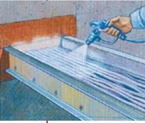
Water-based, spray-applied coating used to provide short term circuit integrity and improved flame spread characteristics for grouped electrical cables.
